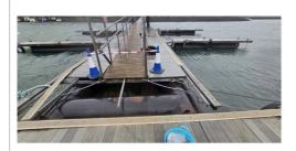
1. Secure Hammerhead Pontoon: Attached the hammerhead pontoon to the main pontoon using heavy chains and shackles to prevent the pontoons from breaking free
